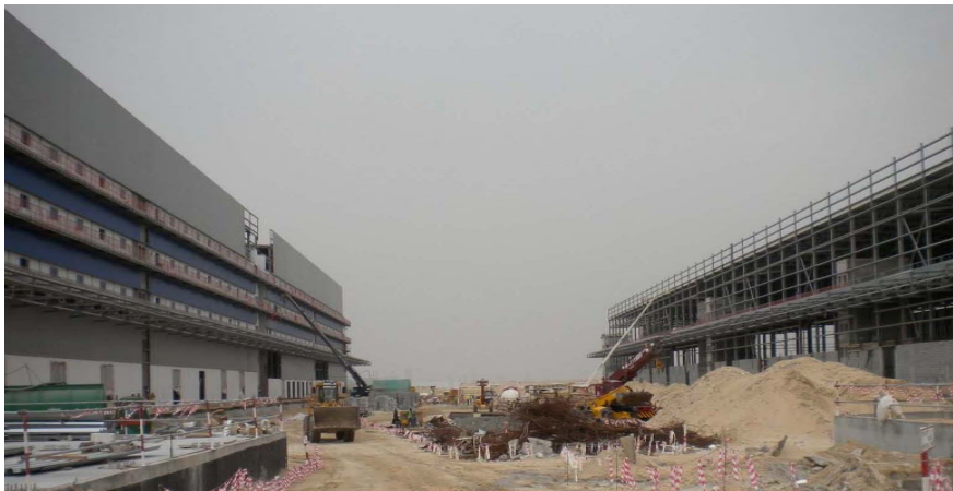
Image 3: Warehouse Complex Under Construction In Dubai
